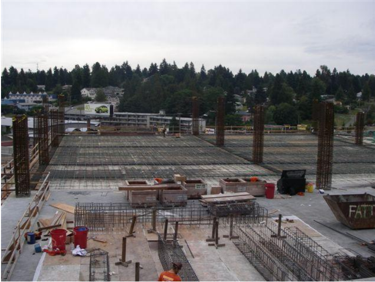
Area F, Level 2 Deck and Column Installation
