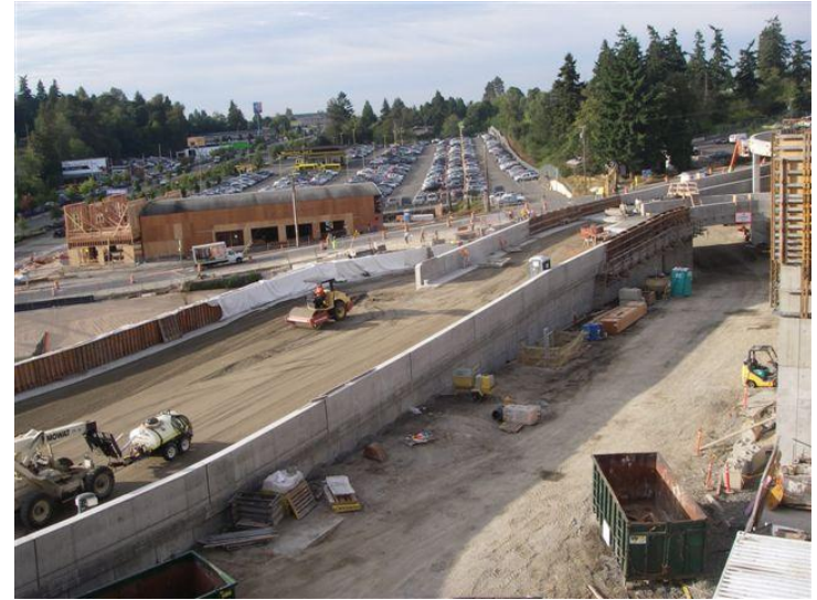
On-Site Roadway Progress
