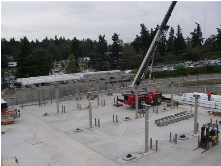
QTA #3 Canopy Installation
