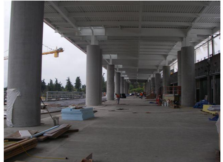
CSB High Roof - East
